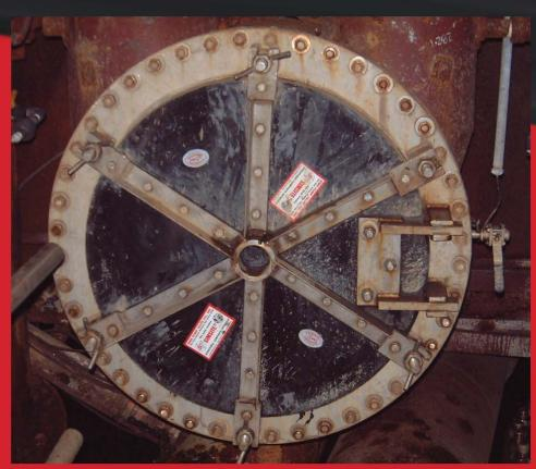
The SIMSITE® Heat Exchanger Door is permanently attached to the heat exchanger and can be easily opened and closed in minutes. This Door as been in Service over 10 Years!
